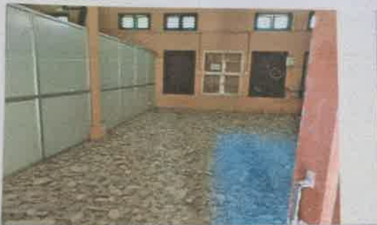
RENOVATION - CANTEN TILE WORK
