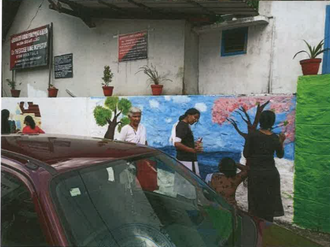
Painting the outer walls of the Excise Range Office, Pala on 03/06/2022.
