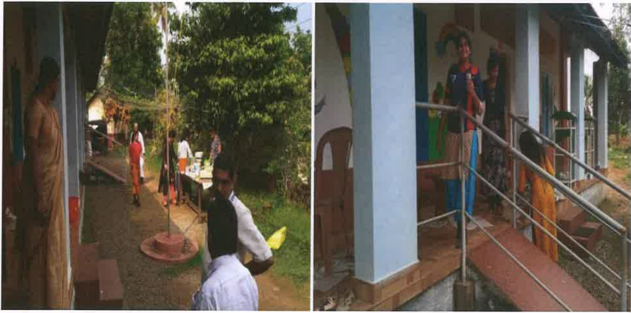
Painted the walls of Govt LPS Arunapuram on 01/04/2022
