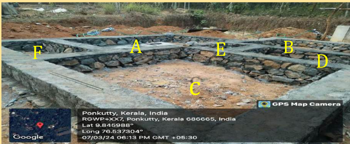
Figure 3: Constructed foundation with the actual plan pointed
