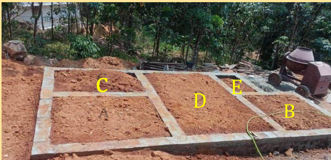
Figure 3: Constructed foundation with the actual plan pointed
