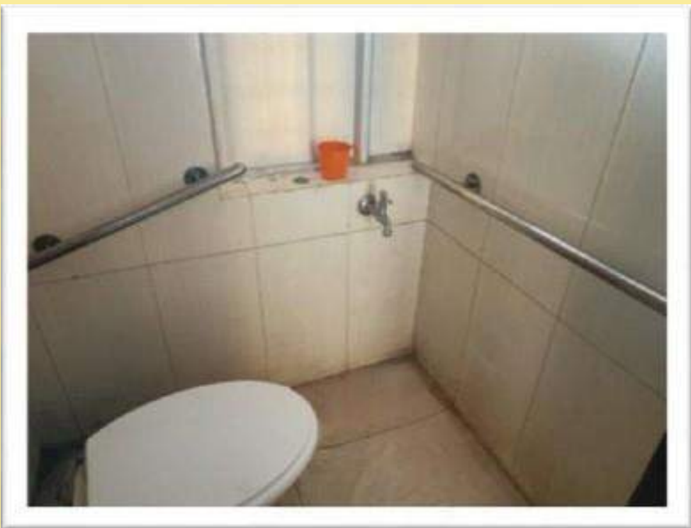
Disabled friendly toilet
